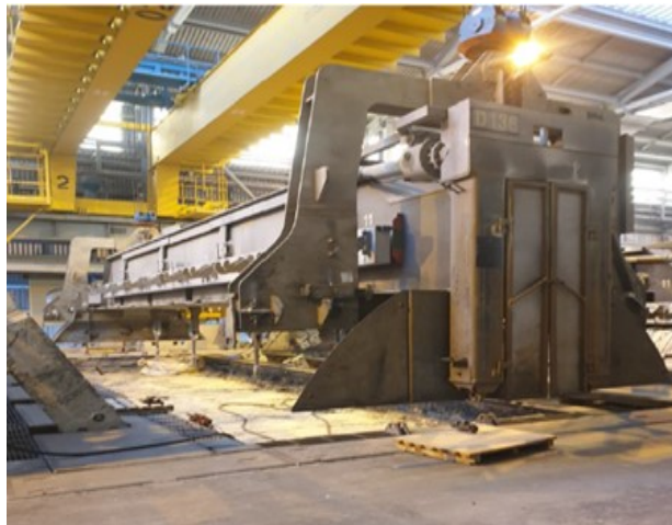
Figure 17. Removal of superstructure.
