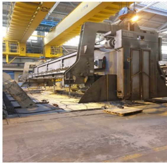
Figure 22. Re-install anode superstructure.
