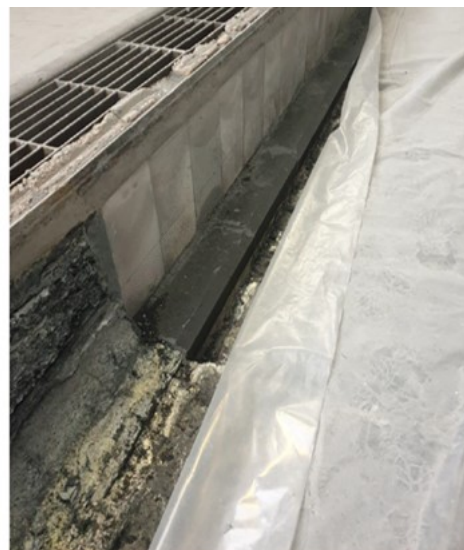
Figure 24. Side wall repair.
