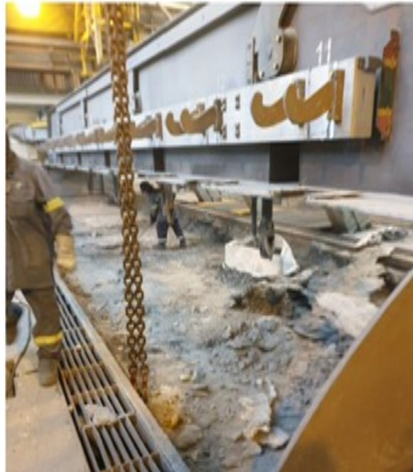
Figure 20. Removal of anodes and metal.
