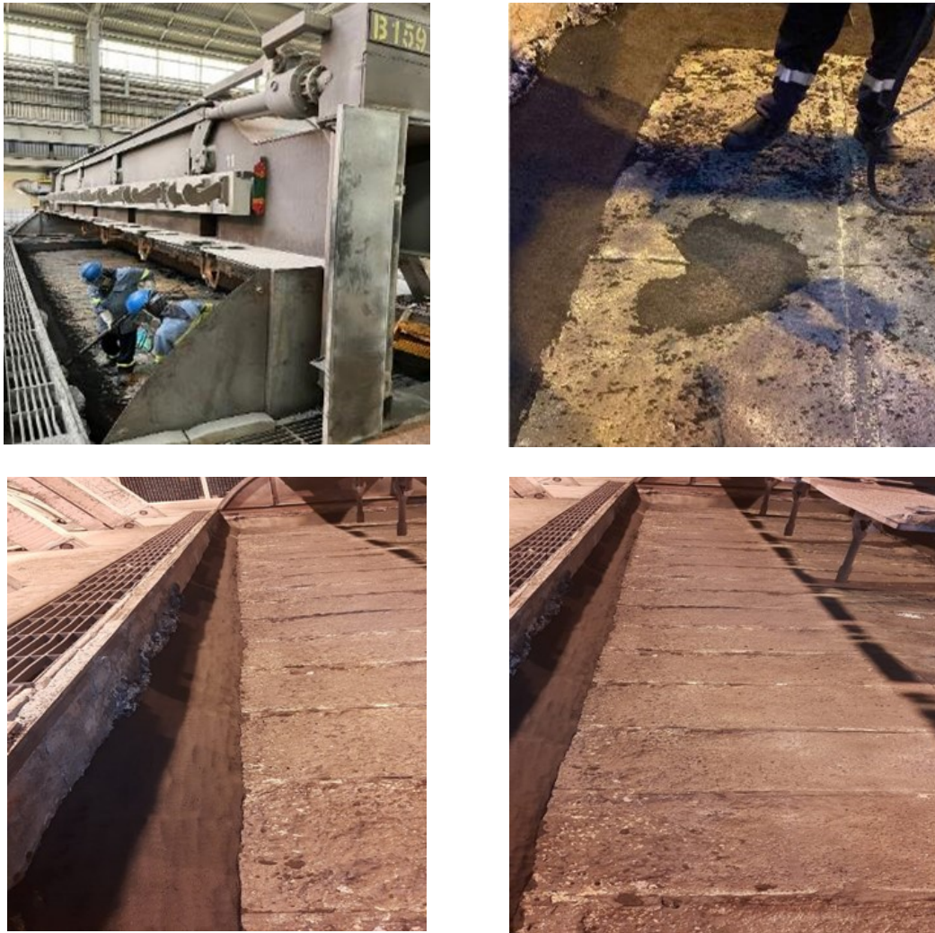
Figure 26. Sidewall and fillet ramming.
